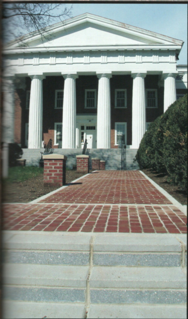
Hall's porch, stairs, and paths have been repaved.
