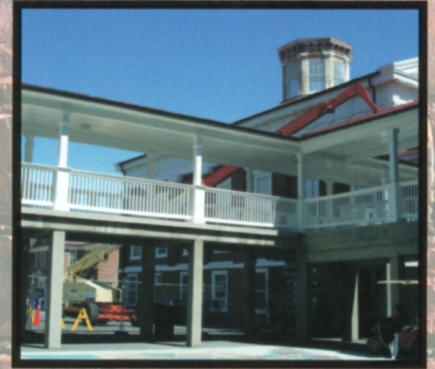
The Chapel and walkways are being repainted.
