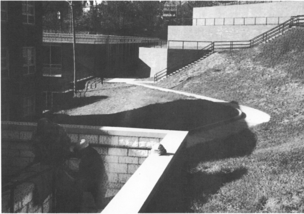
One of the completed projects for handicapped access - sidewalk from Healy Hall to Strader Hall
