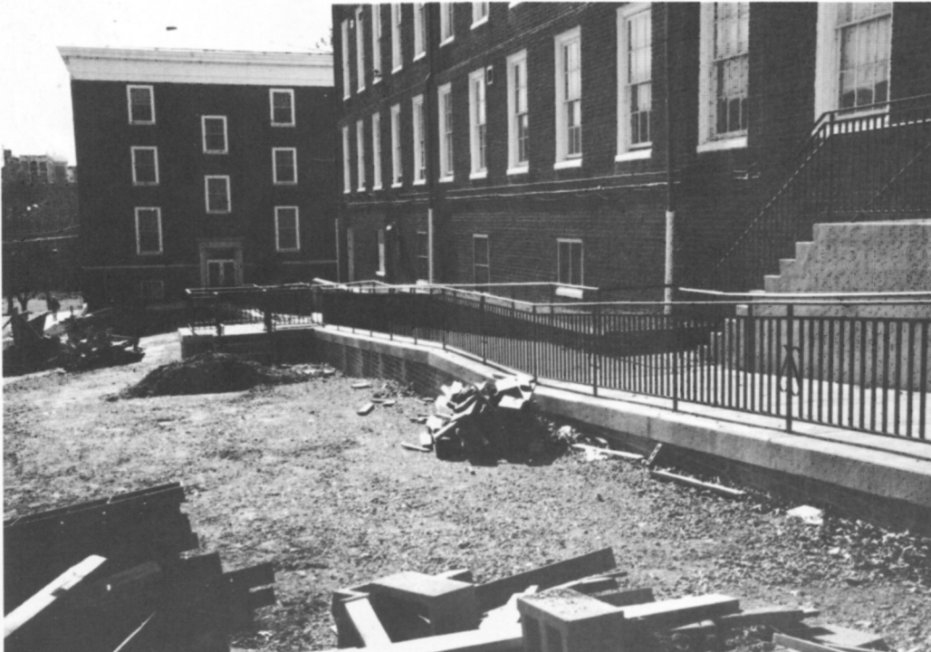
The ramp behind Byrd Hall - nearly completed
