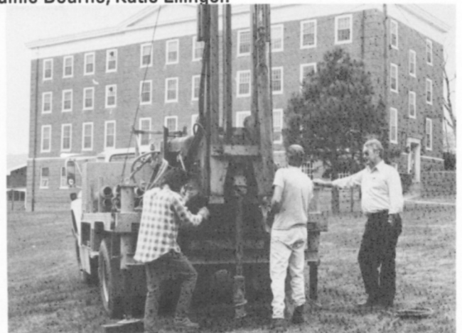
Soil Testing for our future swimming pool.
