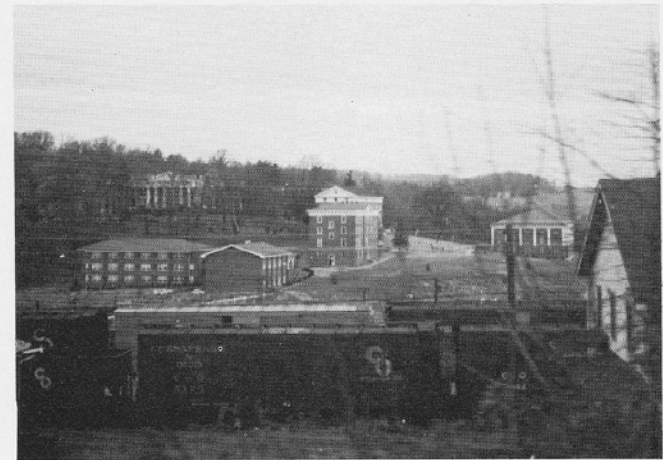
Looking at V.S.D.B. from across the railroad tracks.
