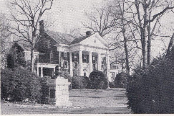
This is the entrance of V.S.D.B. On the left stands the superintendent's home. Through this entrance hundreds and hundreds of deaf students have come and gone.
